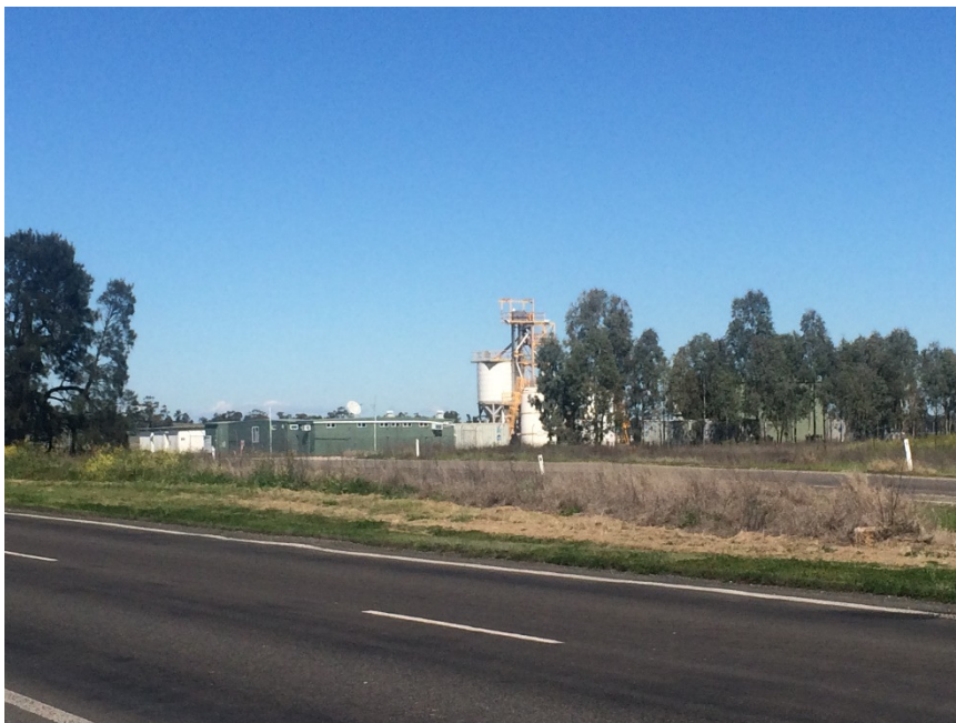
Figure 9 Existing similar facility to the south
